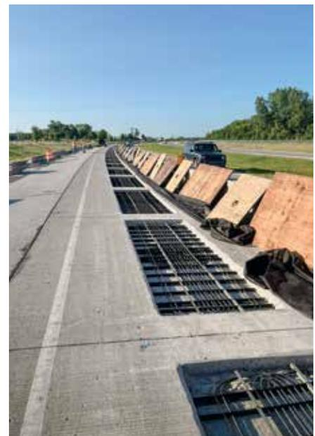
*Construction is in progress on a quarter-mile test bed on U.S. Highway 231 and U.S. Highway 52 in West Lafayette that the team will use for testing how well a patent-pending system designed by Purdue engineers can provide power to a heavy-duty electric truck traveling at highway speeds.*
